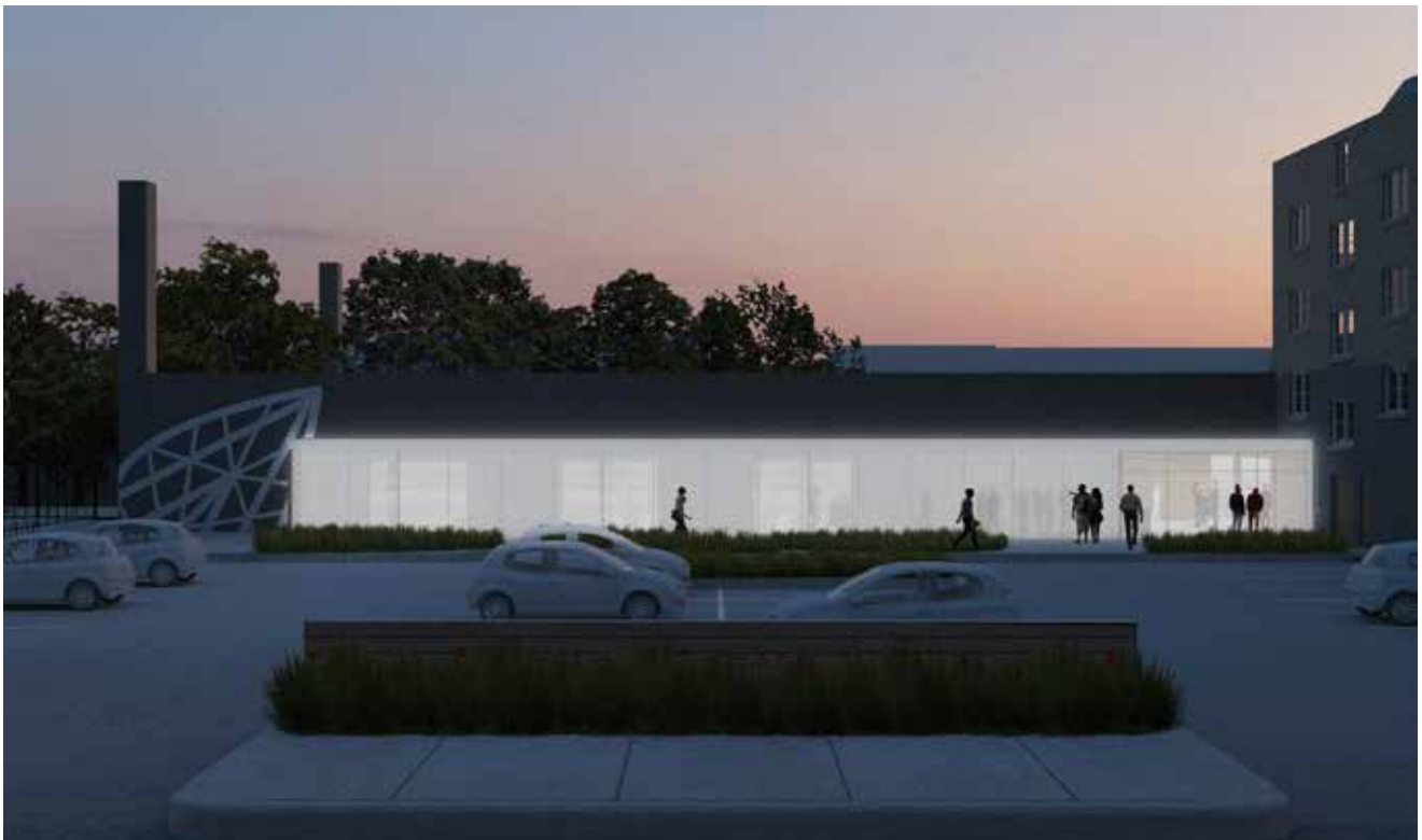
TOP: New facade along W Wells St has large doors that can open up to create an outdoor market on weekends. BOTTOM: Semi-translucent glass creates a bright facade at night that hints at the activity of the facility.
